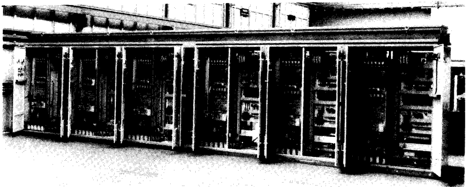
Figure 11-17 Fifteen forced-commutated inverter cubicles for a cement kiln. (Reproduced by permission of Brush Electrical Machines Ltd., England)
